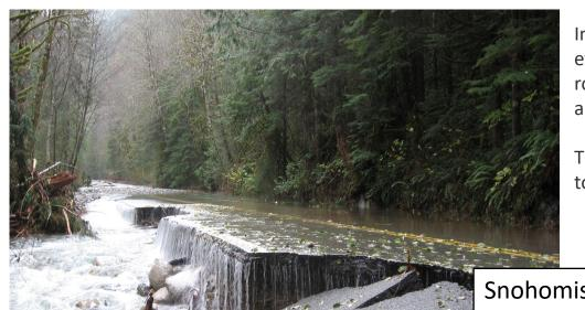
In November 2006, Index-Galena Road was extensively damaged by a major flood event on the North Fork Skykomish River that washed out multiple sections of the roadway. This event resulted in Index Galena Road being closed at MP 6.4, just east and upstream of the Trout Creek Bridge.
