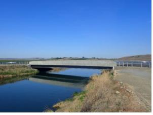
In 2004, rotting timber stringers were detected. A temporary fix was installed in 2017, and federal funds were secured to replace the bridge. This was a Federal Aid Bridge project. A new single span concrete bridge replaced the rotting timber structure. The new bridge is wider, allowing agricultural implements to cross safely.
