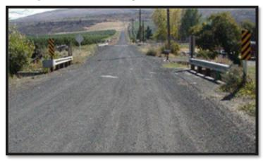
The county was awarded federal funding for bridge replacement, and gained CRABoard funding through the Rural Arterial Program in 2014. The bridge was replaced with a longer and wider precast concrete girder bridge. The farming community is enjoying a stronger, safer crossing that will last a long time.
