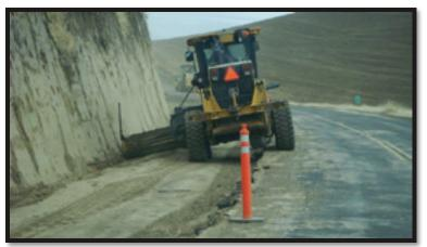
The road was also widened from 22 feet to 28 feet. The intersection between Kellogg Hollow and Whetstone Roads was realigned to intersect at 90°. This work was performed by Thompson Brothers Excavating, Inc., Vancouver, WA
