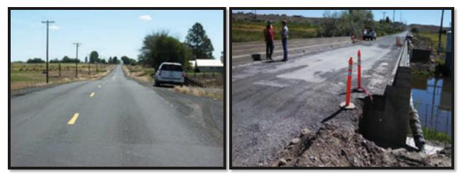
The county improved milepost 0.00 to 3.00 (Stratford Road to M-NE) by doing basic widening from 21 feet to 34 feet on the first mile of the project. The last 2 miles had widening as well as major rebuild of the pavement structure. The public appreciates the wider roadway, the larger radii on intersections, and have noticed the safety improvements for bicyclists.
