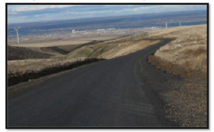
The road had sharp curves and a switch back at the bottom of the canyon with steep grades into and out of the canyon. Side-slopes were steep and guardrails were needed. A fill was built across the canyon eliminating the sharp curves, the switch back alignment, and the steep grades. The new roadway is built to standard width and is an all-weather structure enhanced with guardrails for added safety.
