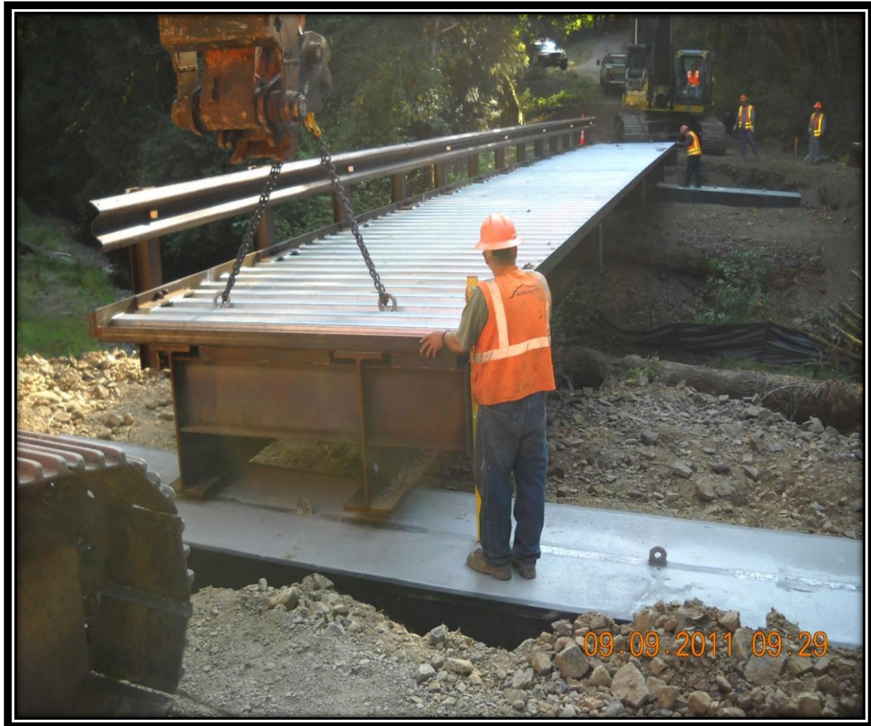
Cowlitz County Road Crew installing a modular steel emergency access bridge intended to provide alternate access during flooding that frequently closes Ostrander Road.
