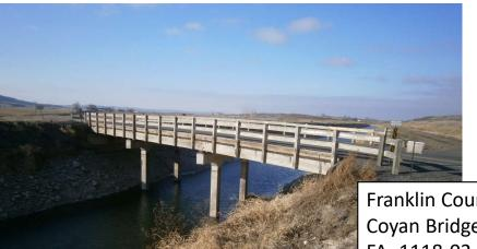
Coyan Bridge #200-9.93 was an 84' three span timber structure constructed in 1955 to span the Columbia Irrigation District's Potholes East Canal. In 2004, rotting timber stringers were detected. A
