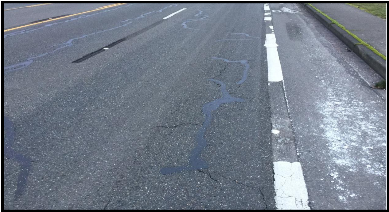
Recessed pavement striping
