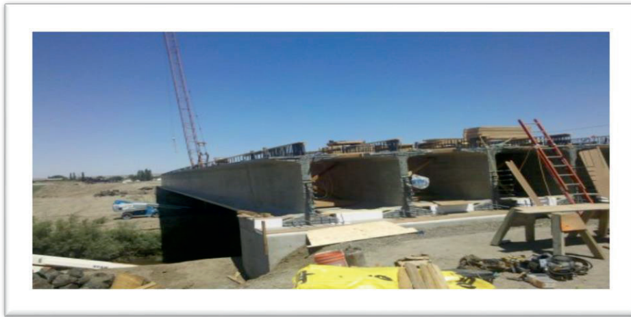
New girders being placed on the new bridge abutments
