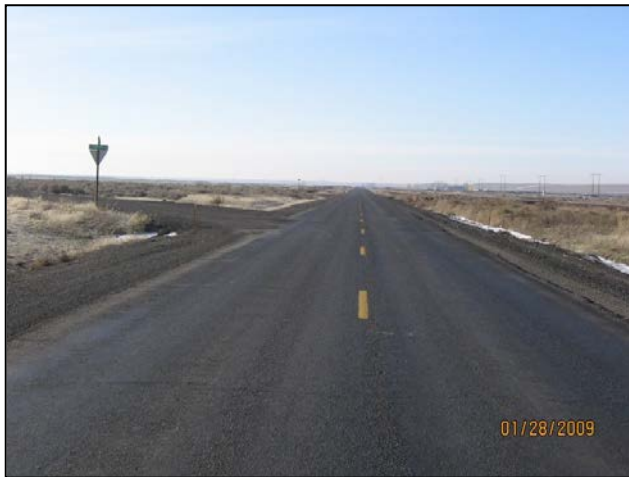
Danekas Road before improvements
