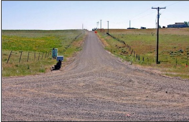
The road in its previous narrow un-surfaced condition.
