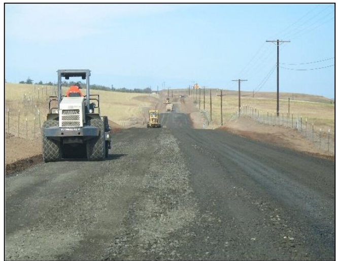
Grading the road to support a wider stronger surface.
