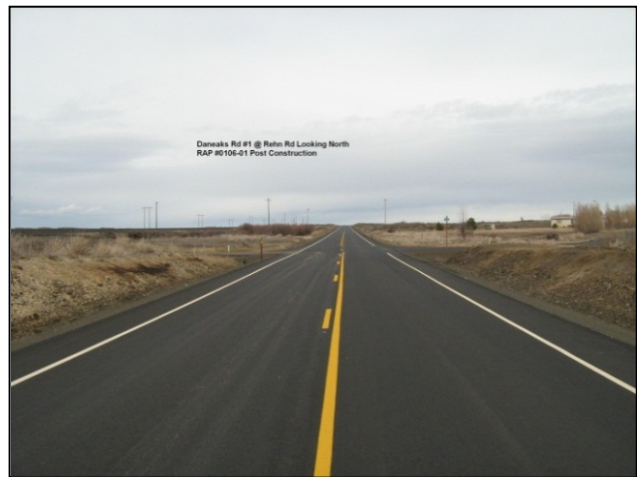
Now built to full width and surfacing standards.
