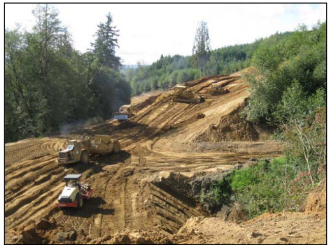
The new roadway requires major excavation.
