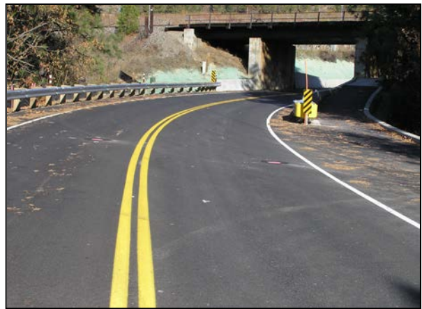
Now a smoother, safer crossing at the bridge.
