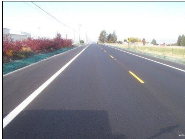
A wider, stronger and safer 4-NE Road.
