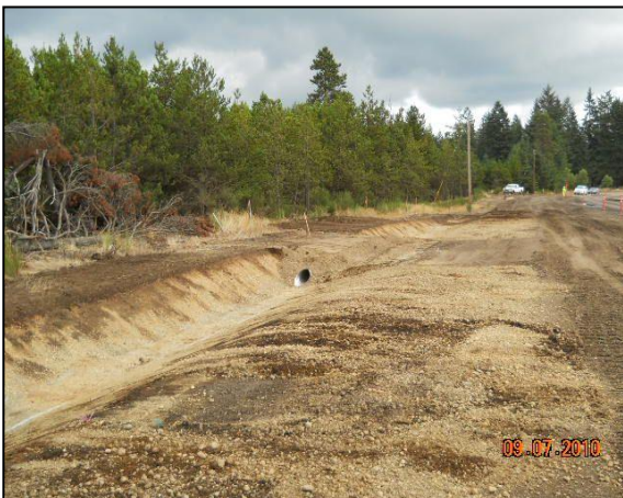
Work commences to widen, add base material and drainage.
