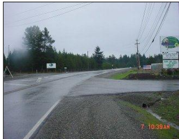
The new and safer Johns Prairie Road.
