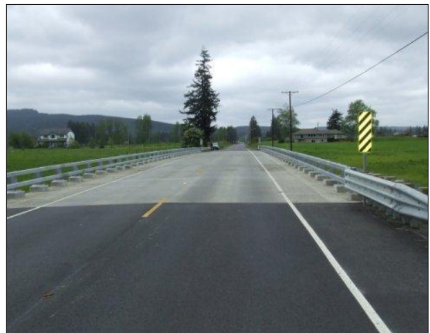
The new bridge, built with a thin, water-shedding profile.
