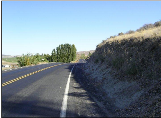
Curves dangerously hid traffic on the old alignment.
