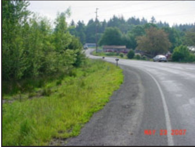
Poor sight distance near beginning of project.
