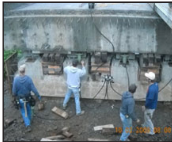
Construction crew jack the bridge to new elevation.
