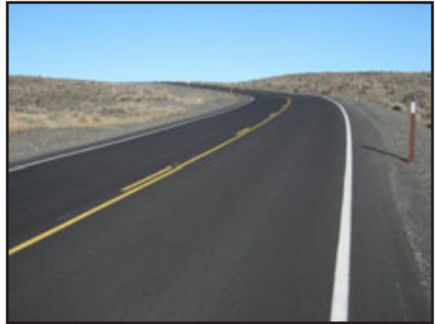
Improved alignment, width and pavement structure.
