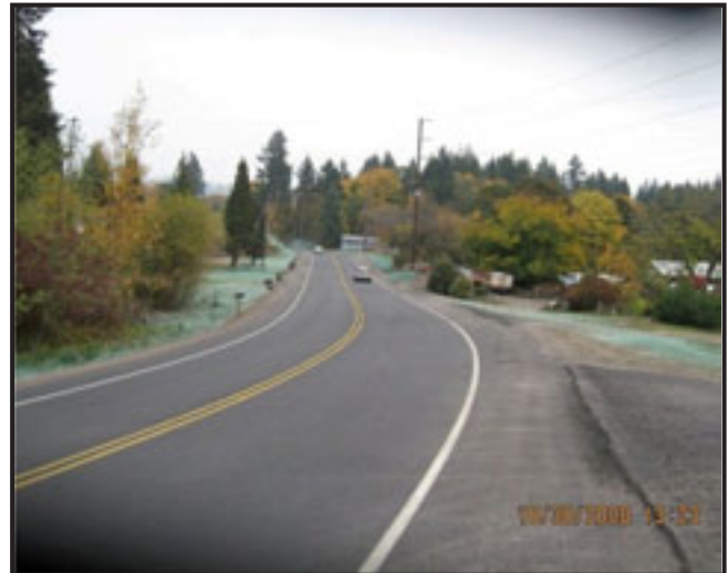
The new roadway is wide open.
