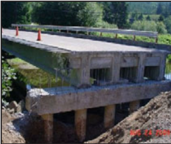
The fix required significant demolition.
