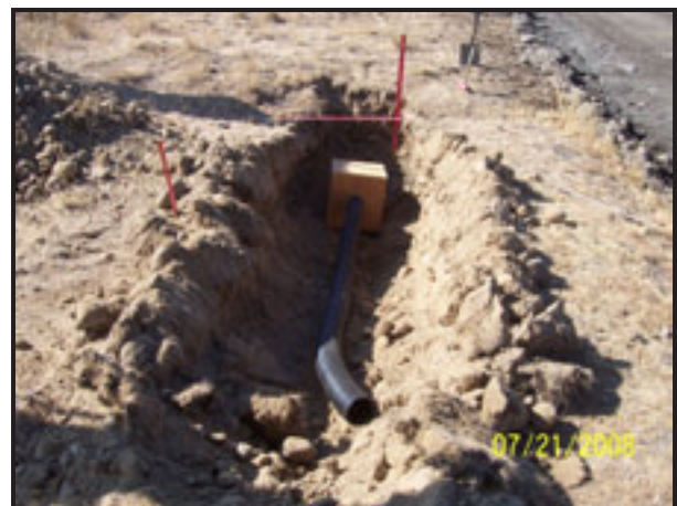
Burrowing Owl Box installed prior to Backfilling.
