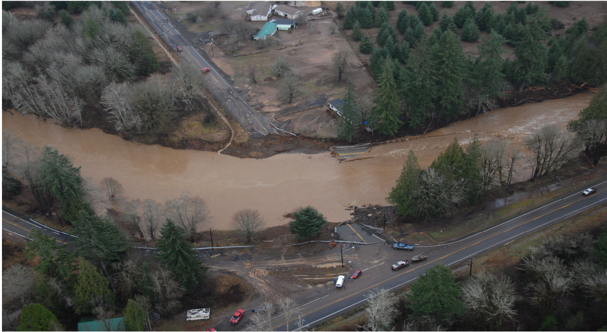
The Chehalis River destroyed Lewis County's Chandler Bridge off Highway 6 near Pe Ell.
